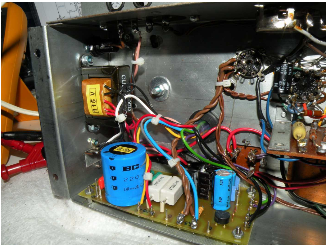
Installation of new PSU board inside the AO-28 chassis.
