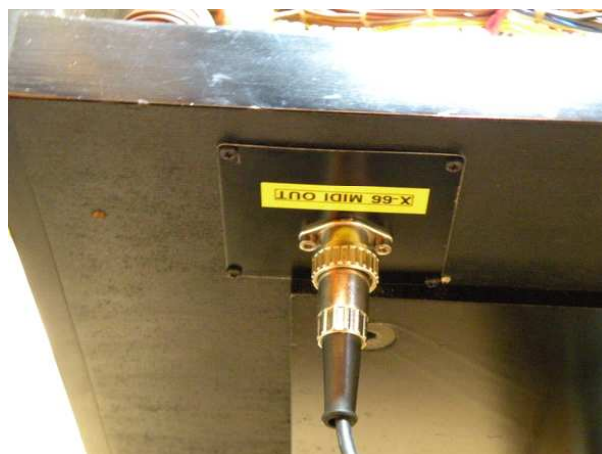
MIDI connection to external units.
